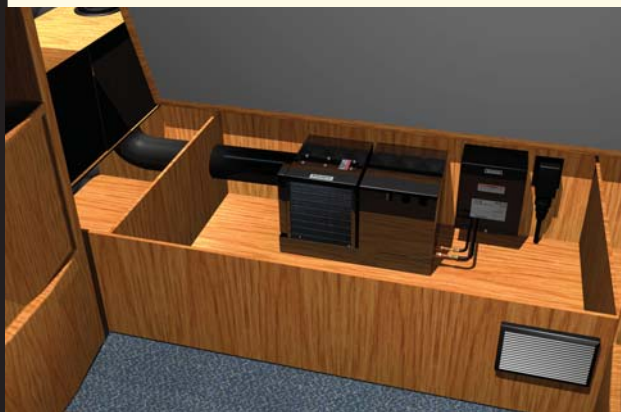
Split system inside unit under bunk.
