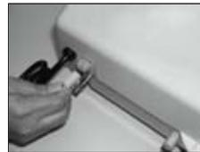
3. Disconnect the humidifier control wires by grasping the nylon connector firmly and pulling straight out.
