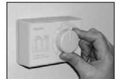
**15.** Test operation. Check for water leaks. Be sure the humidistat is operating properly.
