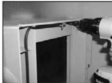
6. Place the mounting frame into the plenum opening so that the frame hooks over the bottom of the opening. Screw the frame to the plenum.
