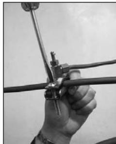
**12.** Tap into the water supply line using the saddle valve provided. Follow the directions on the saddle valve bag.
