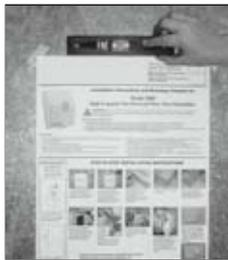
1. Tape the template (this entire sheet) onto the warm air furnace plenum, making sure it is level.
