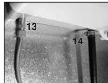
**13.** Connect **copper tubing** from the saddle valve to the solenoid valve. (**Do not use plastic tubing.**) Check for leaks.
