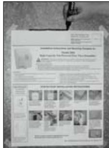
2. Trace around the template. (Cutout size is 13-1/8" wide by 16-1/2" long.) Remove the template. Accurately cut the plenum opening.
