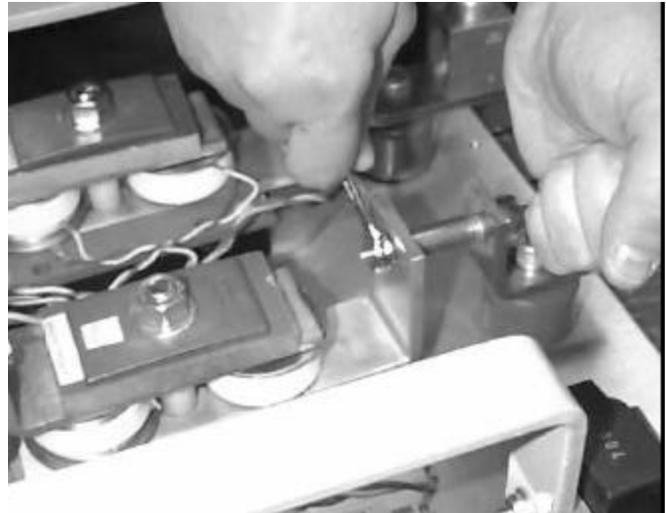
Figure 15. Disconnecting the SCR load side..
