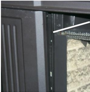
Slide side filler bracket into gap between glass and fire box.
