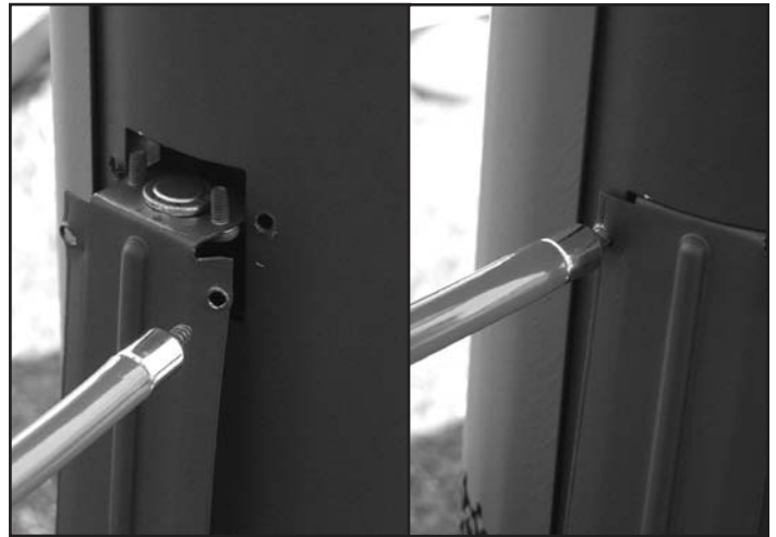
Figure 43: Spill switch installation.
