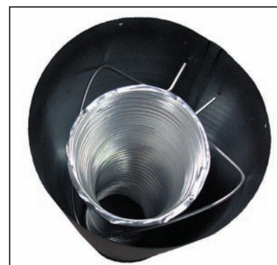
Figure 17: Wire Spacer in Place.
