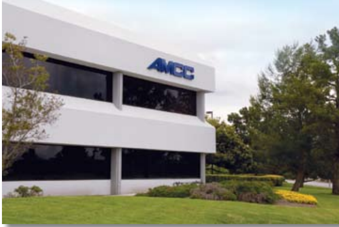
AMCC Headquarters in Sunnyvale, CA
