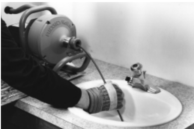
Figure 15 – Push cable down drain line keeping your control hand close to the drain opening
