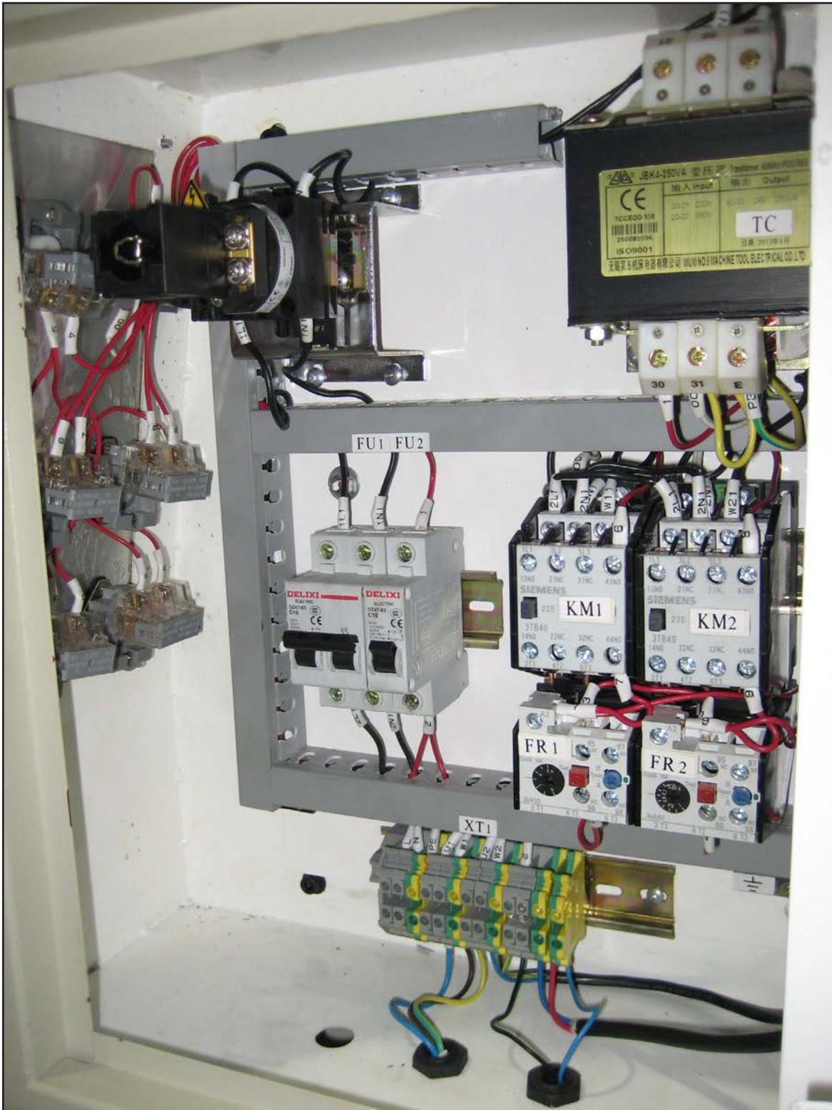
Figure 50. Electrical panel and control panel wiring.
