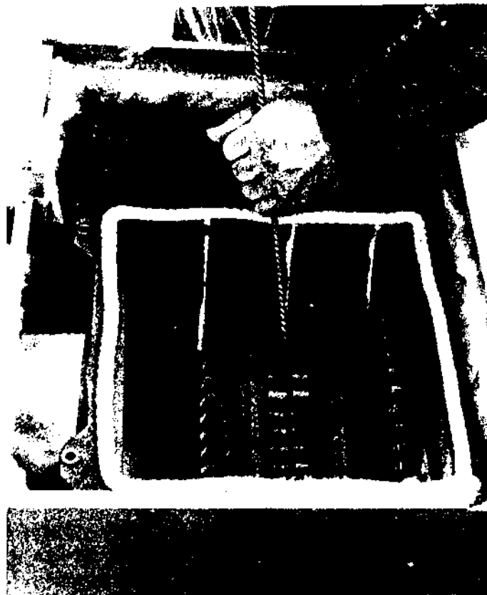
Cleaning Boiler Flueways Figure 3
