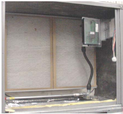
Fig. 22 - Return Air Sensor Operating Position
