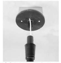
Put plastic cap thru top of the pipe. Run wire thru 1" pipe.
