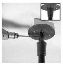
Put 1/4" x 20 screw thru hole and drill in. Add nut for security.
