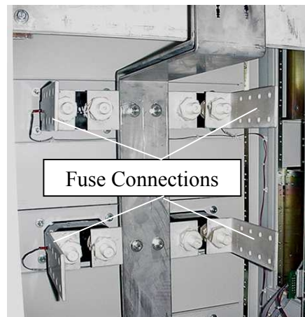
Figure 5-10 Fuse Bay Connections
