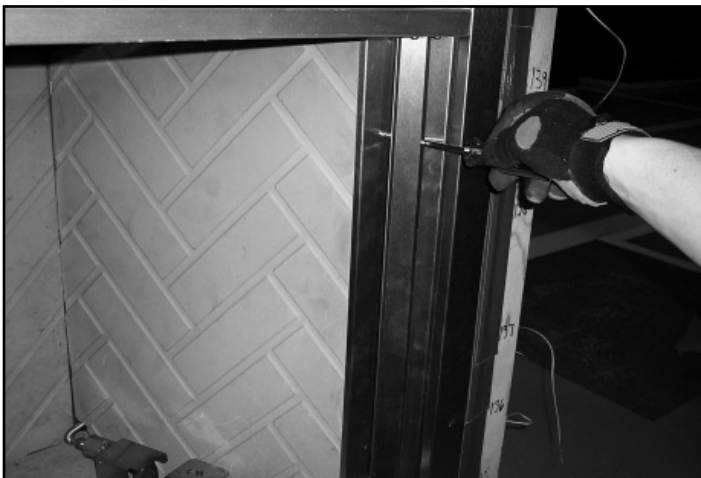
Figure 6.3 Loosen Refractory Retaining Strip
