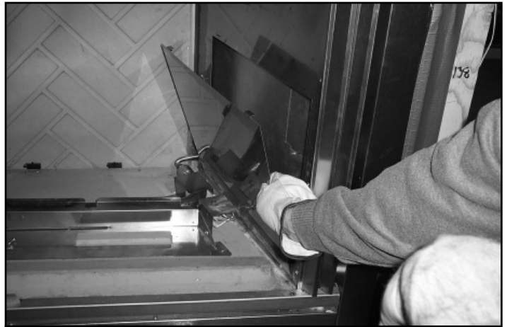
Figure 6.4 Remove Valve Access Panel
