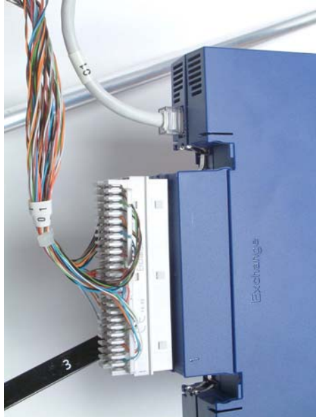
Figure 7 Tie Up and Label the EDGE Connectors
