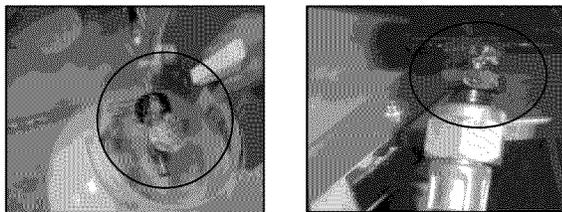
4. If you have a gas connection leak you cannot repair, turn gas OFF at supply tank, disconnect fuel line from your grill and call 1-800-4-MY-HOME or your gas supplier for repair assistance.
