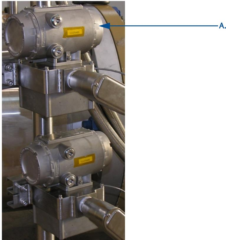
**A. Transmitter Electronics Enclosure end cap**
