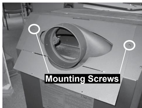
1. After the flue collar has been reversed for a rear vent installation, install the cover plate on the stove with the two screws provided.
