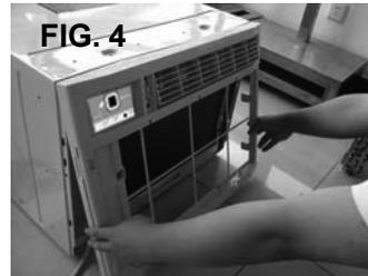
6. Remove shipping crews from top of unit and also on the side by the base if installed.
