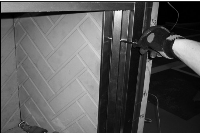
Figure 12.3 Loosen Refractory Retaining Strip
