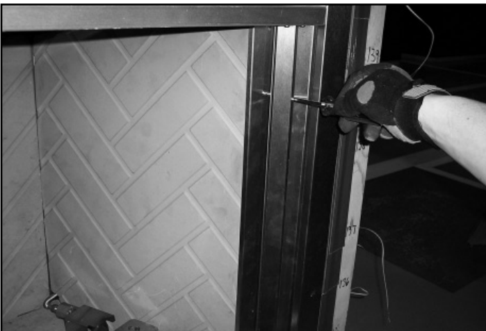
Figure 6.3 Loosen Refractory Retaining Strip
