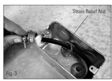
4. Tighten nut to lock strain relief in place. When properly installed, strain relief should look like this (Fig. 4):
