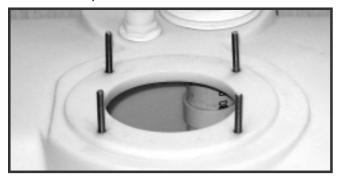
15. Place floor flange seal on studs, aligning the studs with bumps on seat. Note: "THIS SIDE UP" should face upwards.
