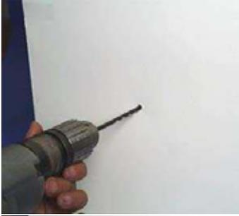
C.4 Interior Wall Mounting: Choose a location on the wall that is directly above the exhaust bulkhead fitting coming out of the back of the sterilizer (See lower picture on page 3). This is the location where the exhaust hose will run through the wall to the outside.
