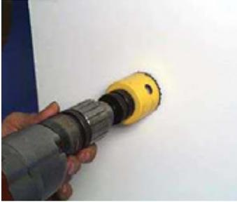
C.5 Using a 2" hole saw bit, enlarge the pilot hole on the interior surface of the wall to 2". Repeat this process on the exterior surface of the wall using the pilot hole as the center point. You should now have a 2" hole through the entire wall.
