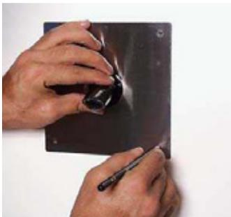
C.13 Exterior Wall Mounting: Slide the exterior mounting plate over the black PVC tubing that extends out through the 2" hole and then mark the four mounting holes.
