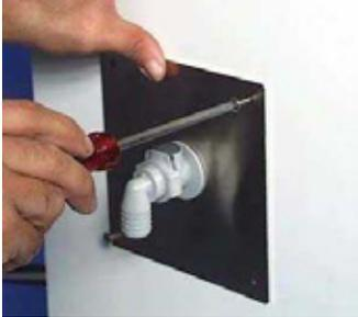
C.10 Secure the interior mounting plate assembly to the interior wall by threading the Phillips screws into the four toggles.
