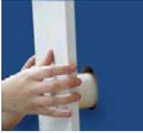
D.2.1 Clean the Mating Surfaces. Remove the mounting plate from the wall and clean the outside surface of the 2" PVC pipe as well as the interior surface of the tube extending from the back of the plate with rubbing alcohol and allow to dry.
