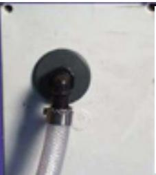
D.3.6 Move the sterilizer into its permanent location and then stretch the clear braided PVC tubing up to the 90 degree wall mount fitting. Allow for an extra inch or two and cut to length. Slip a stainless steel hose clamp over the tubing and then push the tubing as far as it will go onto the 90 degree hose barb connector. Secure the PVC tubing with the second stainless steel hose clamp.
