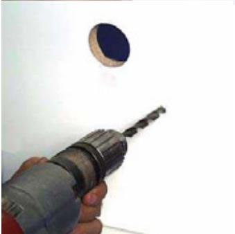
C.7 Remove the interior wall plate assembly and drill the four toggle mounting holes using a 3/8" (.95 cm) bit.
