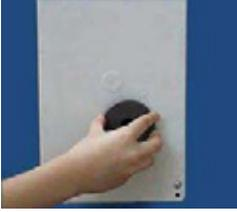
D.3.3 **QUICKLY** press the adaptor all the way into the hole. The glue acts as a lubricant, so it will easily slide in. **NOTE: There can be no delay in sliding the adaptor into the hole after applying the glue. The glue dries in seconds and any delay will prevent correct placement.**
