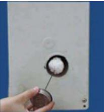
D.3.2 Apply a thin film of PVC glue to each of the mating surfaces, including the inside of the 2" PVC pipe.
