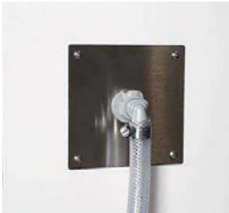
C.12 Move the sterilizer into its permanent location and then stretch the clear braided PVC tubing up to the 90 degree wall mount fitting. Allow for an extra inch or two and cut to length. Slip a stainless steel hose clamp over the tubing and then push the tubing as far as it will go onto the 90 degree hose barb connector. Secure the PVC tubing with the second stainless steel hose clamp.
