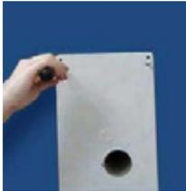
D.2.4 Secure the Mounting Plate to the Wall. Screw the mounting plate to the wall using the original 4 small screws.
