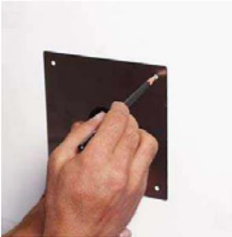
C.6 Take the Interior wall plate assembly (marked "D") with the 90 degree elbow attached and insert the black tube through the hole to the outside. Center the tube inside the 2" diameter hole and mark the location of the four plastic toggles.
