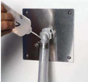
C.21. While the pumps are running, squirt or pour a small amount of the soapy water solution onto the visible connections. If you see any air bubbles that are growing larger, this is an indication that air is escaping from the fitting. Tighten the stainless hose clamps further until the bubbles stop getting larger.
