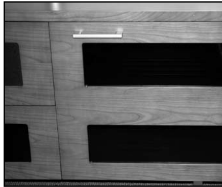
CORRECT! Door is sitting squarely and evenly spaced on tops and sides.
