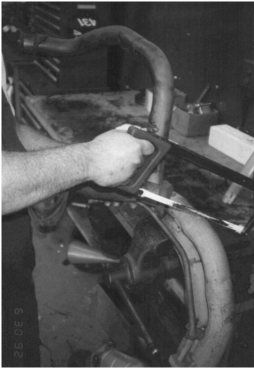
Figure 4a After marking pipe to be cut, clamp securely, then cut with hacksaw
