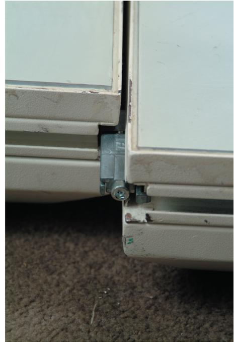
4. To remove the connector, loosen the allen screw and slide the two dance floors apart.
