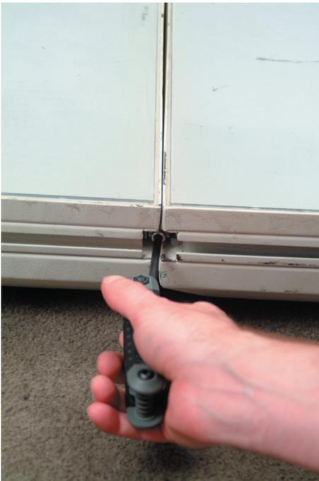
3. Once the connector is pushed all the way in, use a 5mm allen wrench to tighten the connector.
