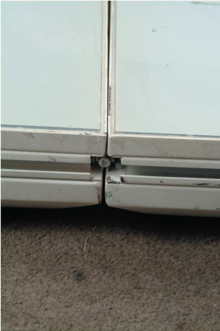
2. Slide the connector until the metal tab stops it from going any further.
