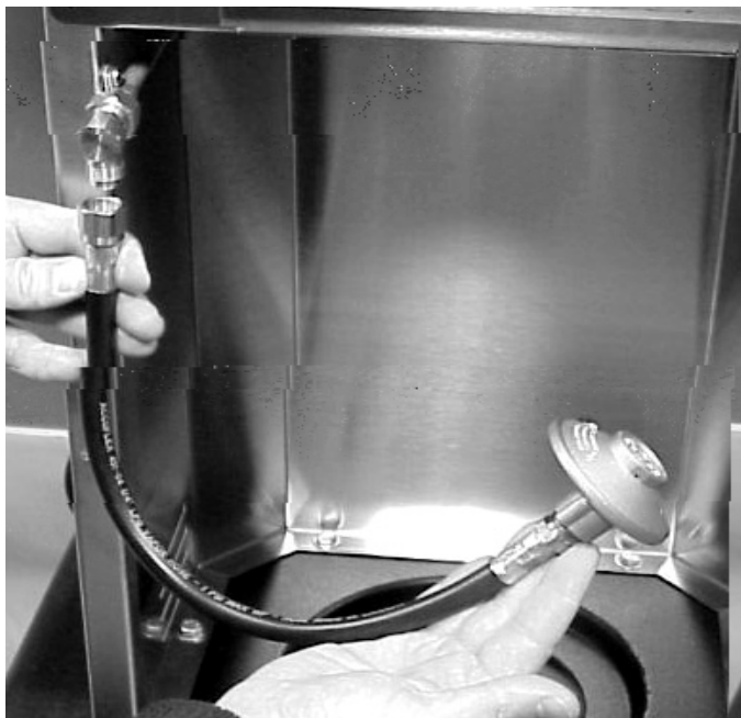
Figure 15 LP Hose/Regulator Connection
