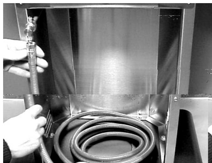
Figure 16 Natural Gas Hose Connection
