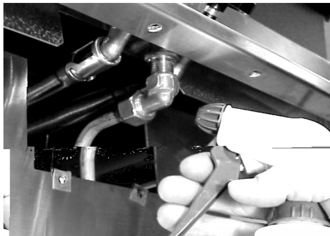
Figure 17 Leak Checking the Valve Connection
