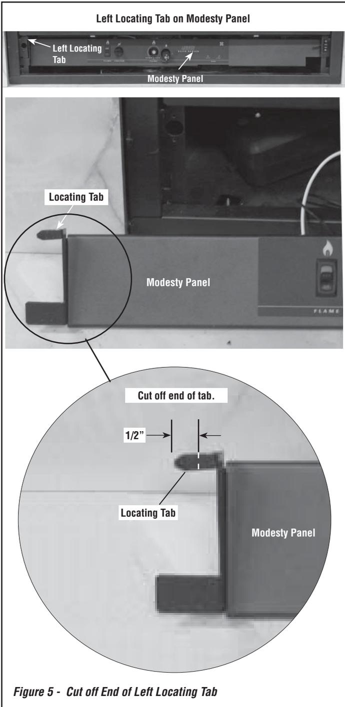
**Figure 5 - Cut off End of Left Locating Tab**
