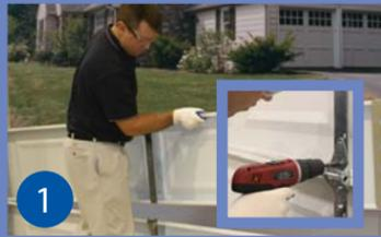
1 Stack the Sections & Attach Hardware
