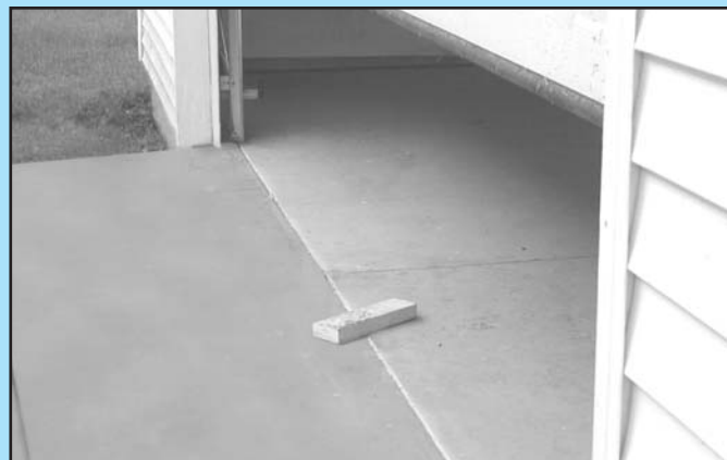
FIG. 6-5 2 x 4 under center of door opening.
