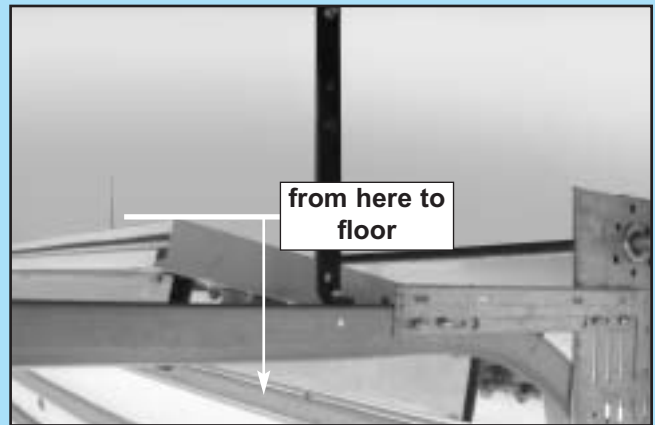
FIG. 2-1 Finding highest point of travel (sectional).
