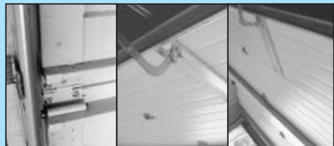
FIG. 2-6 Examples of door bracing.
