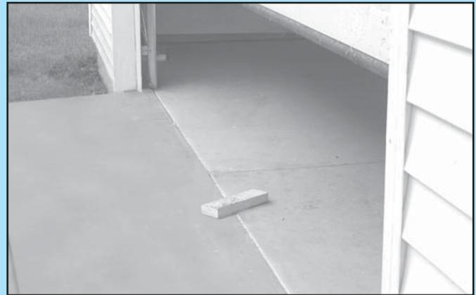
FIG. 6-6 2 x 4 under center of door opening.
