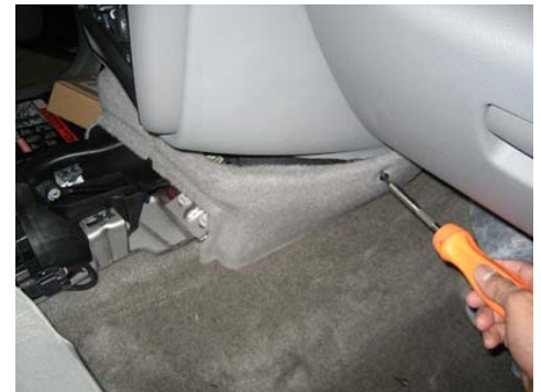
Remove front trim to aid in running additional wiring.
