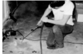
Clean out Debris
