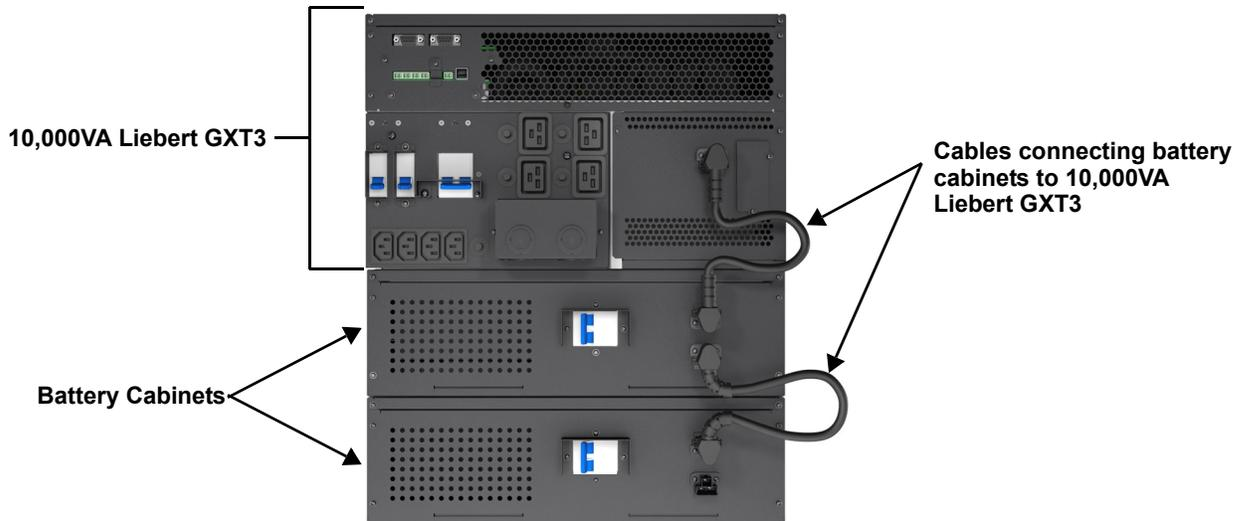
1. Visually inspect the external battery cabinet for freight damage. Report damage to the carrier and your local dealer or Emerson® representative.
