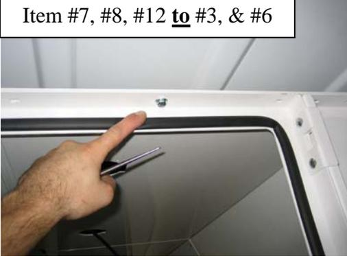
Continue around the entire kit bolting all **Ceiling** pieces to **Bulkheads** and **Doorframes** using 1/4 x 3/4" carriage bolts, washers, and serrated nuts
