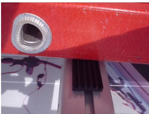
Position rubber pad (T) under ladder rail on opposite side of clamp.
