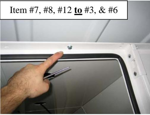
Continue around the entire kit bolting all **Ceiling** pieces to **Bulkheads** and **Doorframes** using 1/4 x 3/4" carriage bolts, washers, and serrated nuts
