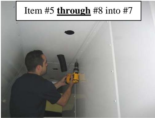
Pre-drill through **Ceiling** sections, (using **Divider** as a template), with 3/16" drill bit and attach using 1/4" x 1 1/2" hex head lag bolts
