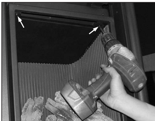
Figure 12: Firebox Baffle Screws Removal.
