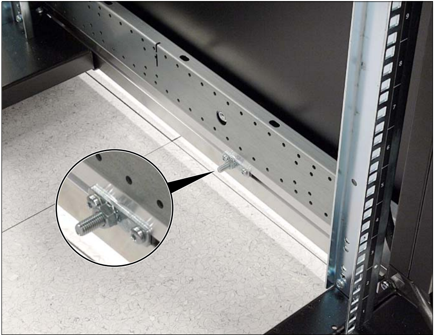
Figure 73: Grounding screw
