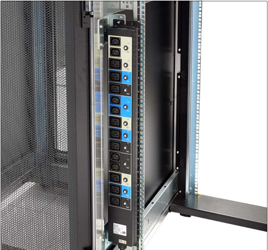
Figure 51: 32 A three-phase 15-way socket strip mounted in a 700 mm wide symmetrical rack
