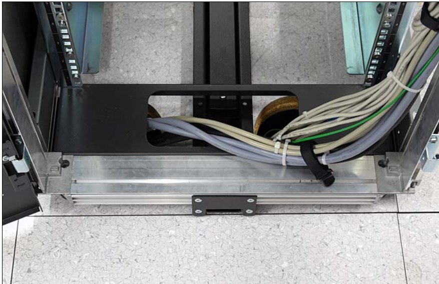
Figure 15: Cable routing through the false floor
