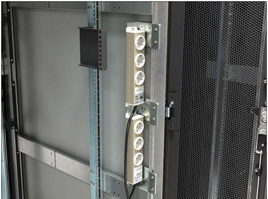
Figure 67: Socket strip extension 3 safety plugs and assembly mounted 2x in a 700 mm wide asymmetrical rack
