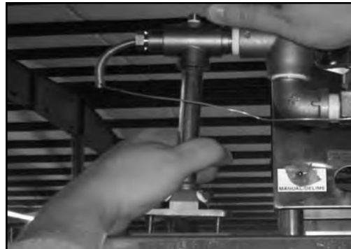
Lifting the rinse injector to make room
