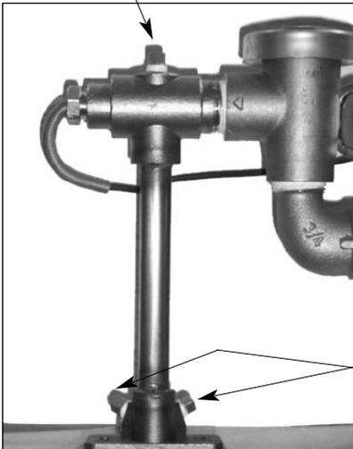
The 1/8" brass plugs on the incoming plumbing rinse injector may be removed to install sanitizer and rinse aid injection fittings.
