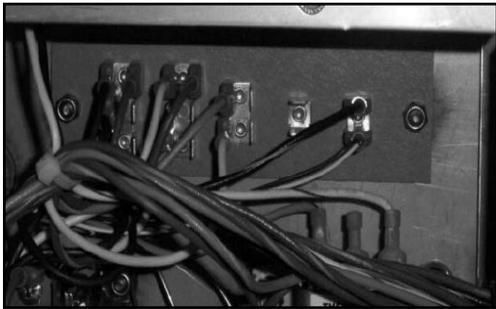
Terminal board inside the heater box
