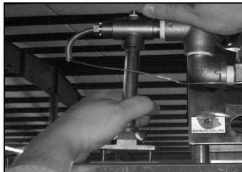
Lifting the rinse injector to make room
