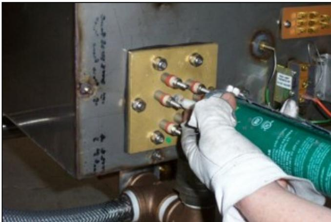
Applying silicone to the heater well
