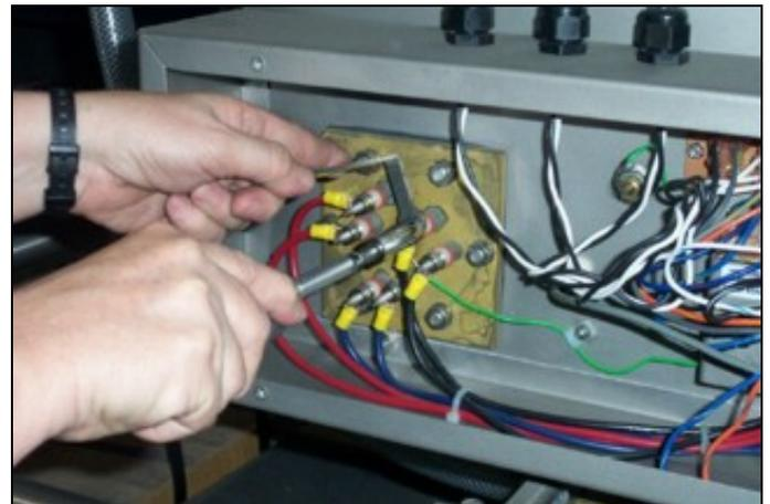
Tightening the nuts holding the power lines
