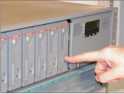
Slide the locking catch to the right to allow locking handle to spring open.
