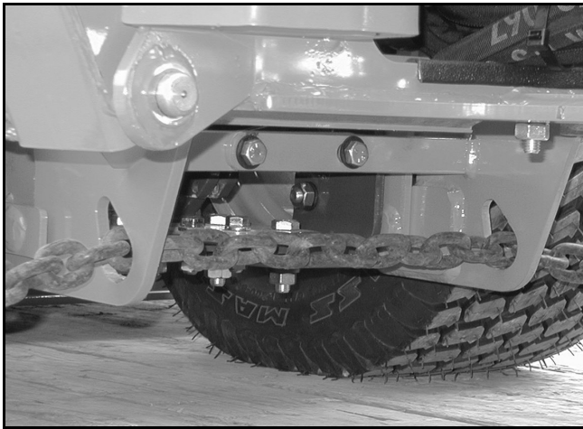
Figure 12. Backhoe Tie Down Location
