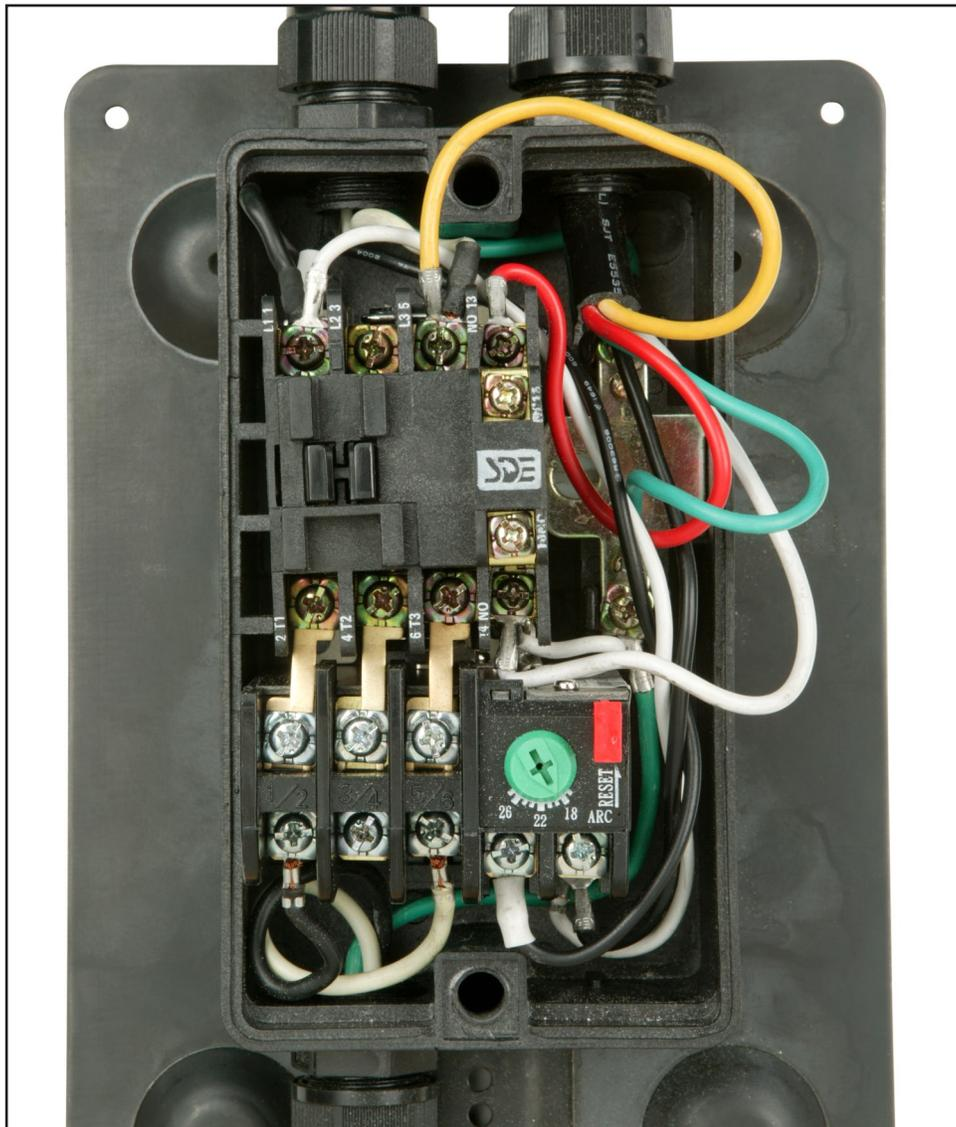
Figure 75. Magnetic switch wiring.
