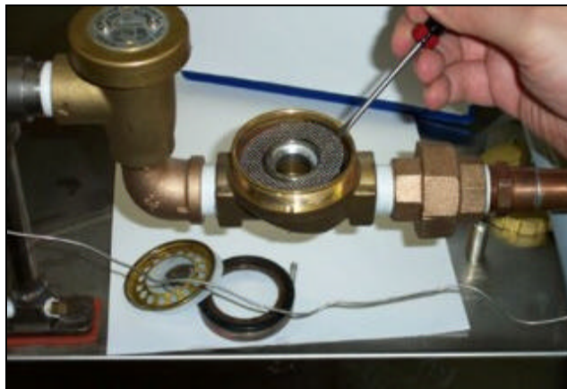
Removing the mesh strainer screen
